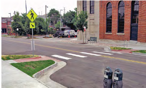
Curb Extension "Bump Out"
